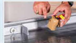
Limit Switch Installation
